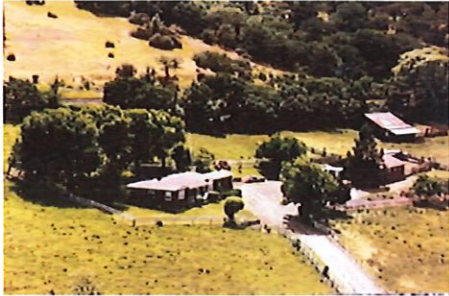
The Existing Farmhouse and Barn
